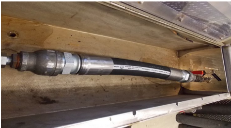
Assembly prior to heat soak and pressurization
